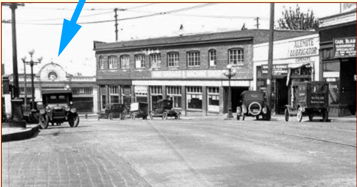
STREET VIEW OF LOCATION #4 (PHOTO BELIEVED TO BE TAKEN IN 1921)
