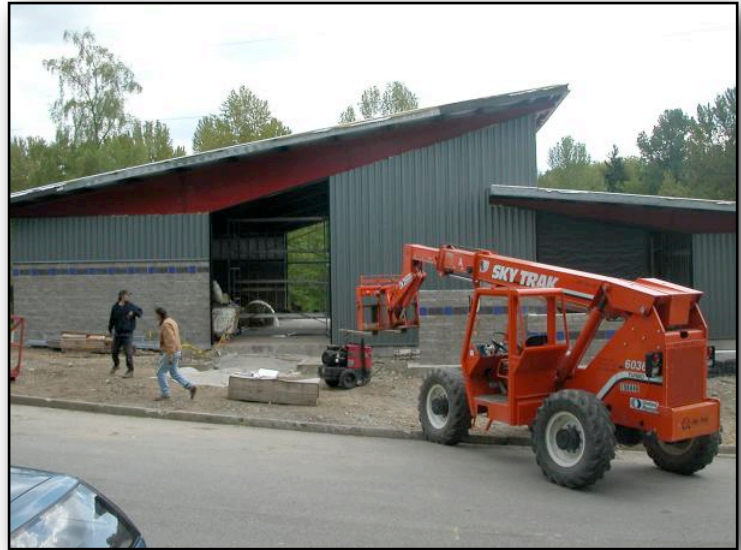
CONSTRUCTION OF THE FACILITY IN 2003
