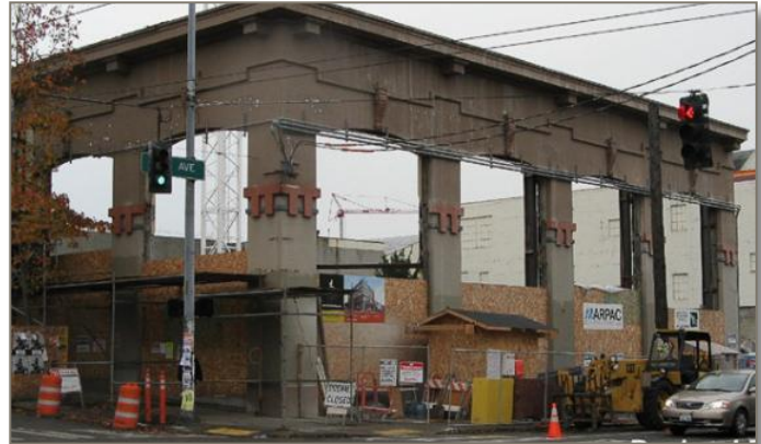
GUTTED KOLAR'S BUILDING DURING THE CONDO CONVERSION IN 2009
